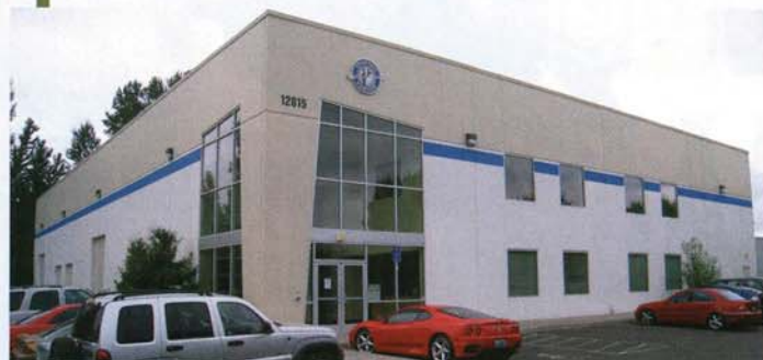
Courtesy Vending custom built its headquarter building to utilize a variety of green and sustainable concepts such as extensive glass to light the interior spaces during the day.
